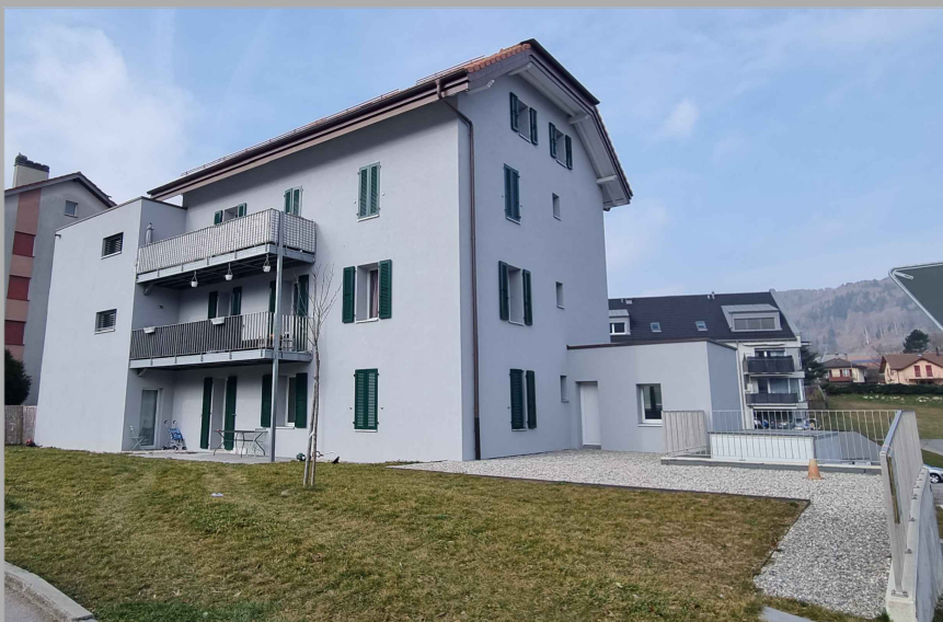
MOUDON - VD - BALUSTRADES - OSSATURE BALCON
